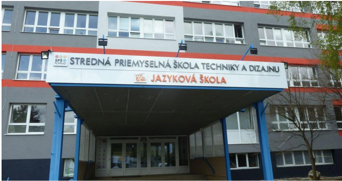
Entrance to the main branch of the Jazyková škola Poprad.
